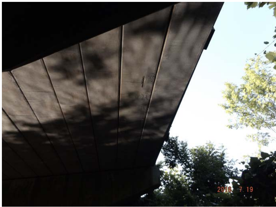
SPAN 2 - BEAM B - REBAR SPALL
