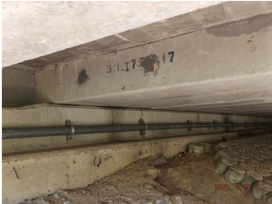
BRIDGE # - SPAN 1 - RIGHT
